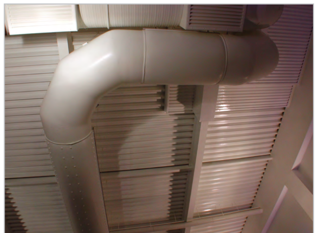
Sample installation: 90° bends in two directions
