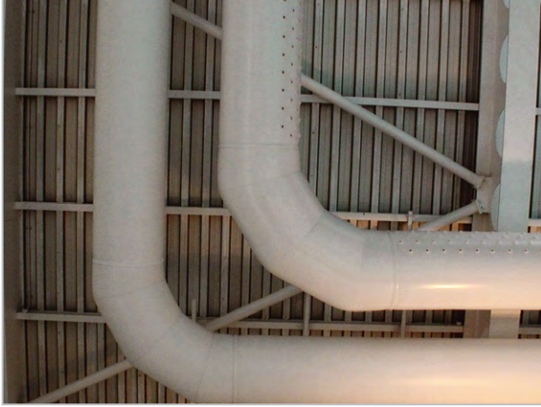
Sample installation: 90° bends
