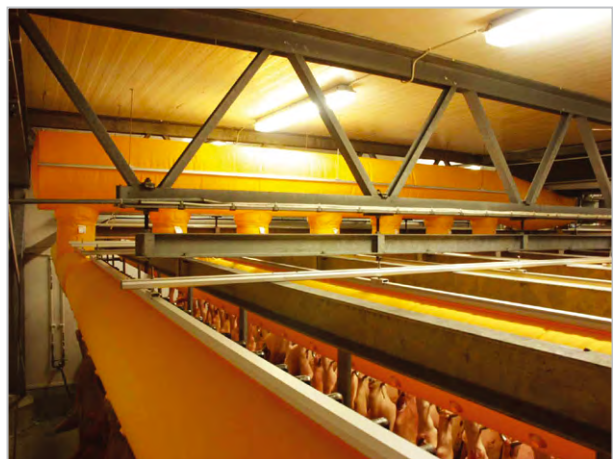
Equalising room: Uppsala, Sweden
