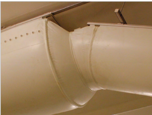
Sample installation: D-duct with a reduction and offset
