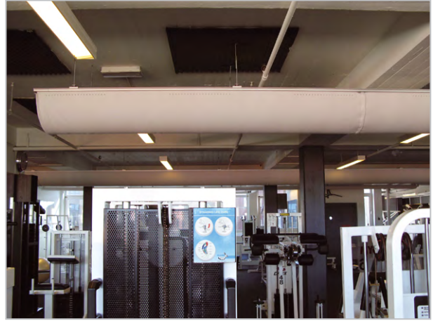
Sample installation: Suspended D-duct
