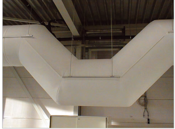
Sample installation: Offset with 45° elbows
