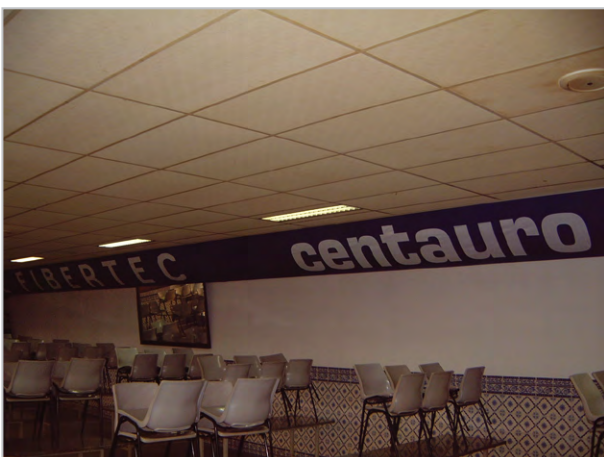
Sample installation: ½D-duct with a printed logo
